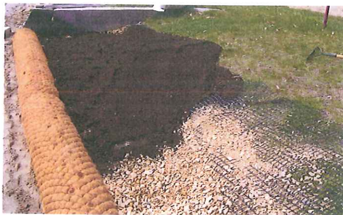
Figure 4.29. Gravel and topsoil fill reinforced with vinyl geoweb. (Photo: landowner.)
