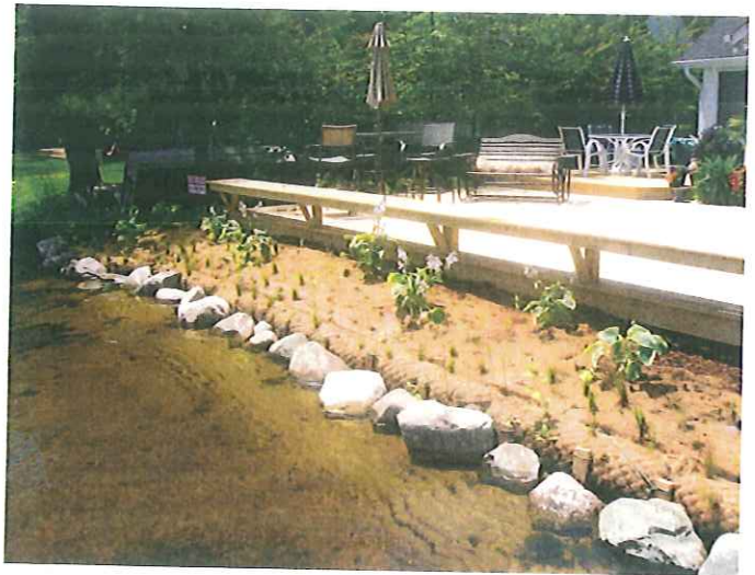
Figures 4.19. "After" picture. Erosion control included a mix of soft- and hard-armoring techniques to stabilize the shoreline and offer protection from erosive forces. (Photo: Jane Herbert.)
