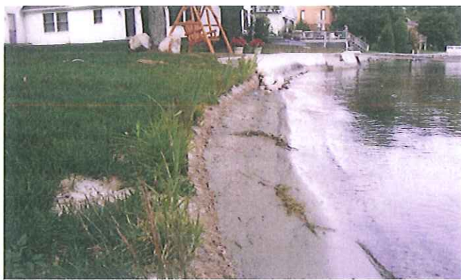
Figure 4.32. Sand deposited behind a log that was placed below the OHWM. (Photo: Courtesy of landowner.)
