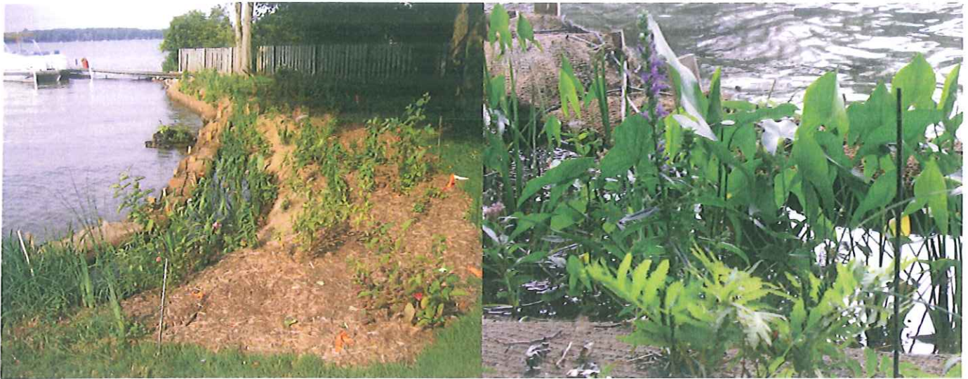
Figure 4.11. Bioengineered erosion control and buffer strip of native wetland and aquatic plants at seven weeks after installation. Gull Lake, Kalamazoo County, Mich. (Photos: Jane Herbert.)
