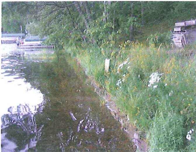
Figure 4.12. Undercut bank stabilized with a biodegradable log (brush bundle) and plantings. (Photo: Jane Herbert.)
