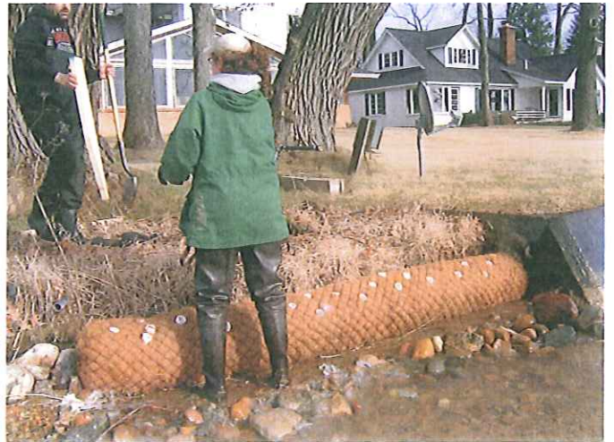
Figure 4.21. Coir log installation, March 2008. (Photo: Jane Herbert)
