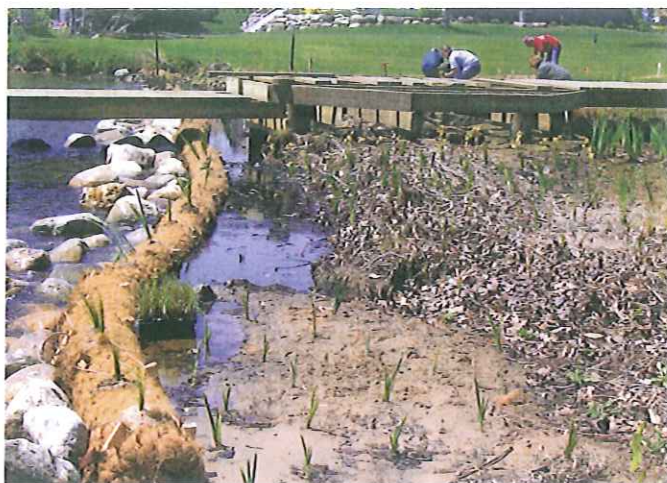
Figure 4.26. Planting native wetland plants in and behind the coir logs (May 2005). (Photo: JFNew.)
