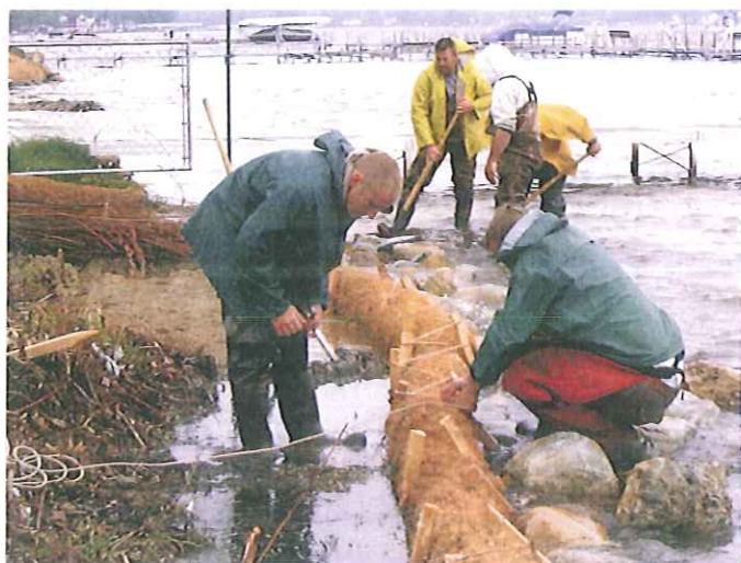
Figure 4.25. Lashing down staked coir logs with nylon rope (foreground). Previously placed stones are being rearranged by hand. (Photo: JFNew.)
