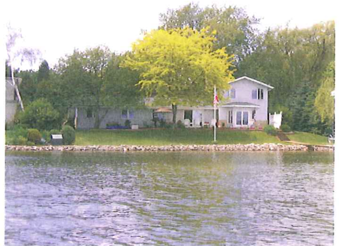
Figure 2.7. Rock riprap erosion control on developed lakefront property. (Photo: Jane Herbert.)
