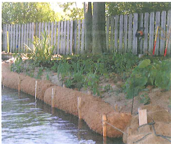
Figure 6.1. Recently installed natural shoreline landscape (Photo: Robert Schutzki.)
